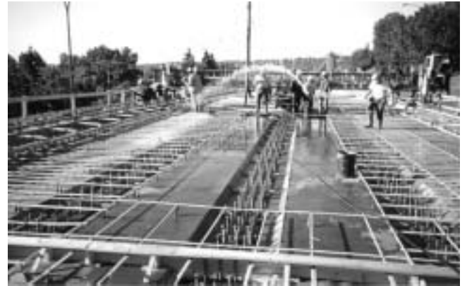
Fig. 2.2—GFRP bars installed during the construction of the Crowchild Bridge deck in Calgary, Alberta, Canada, in 1997.
