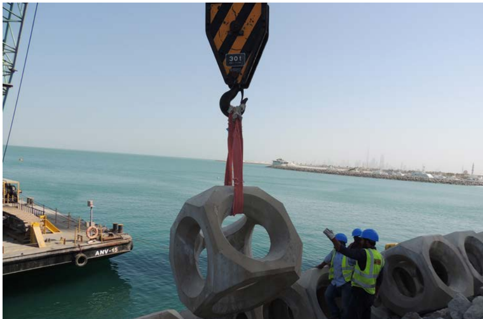
GFRP products were used in the construction of Dubai’s Burj Al Arab Hotel. These included SHED wave energy dispersion units, made with white concrete, with octagonal and circular layers of mateenbar reinforcement. Photos courtesy of Pultron Composites.
